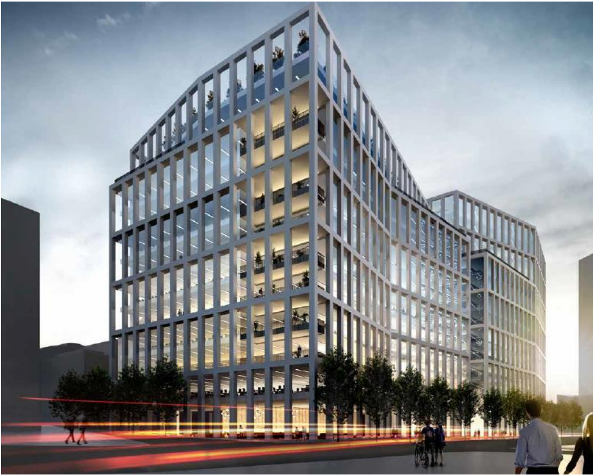
View from Medlock Street Looking North
